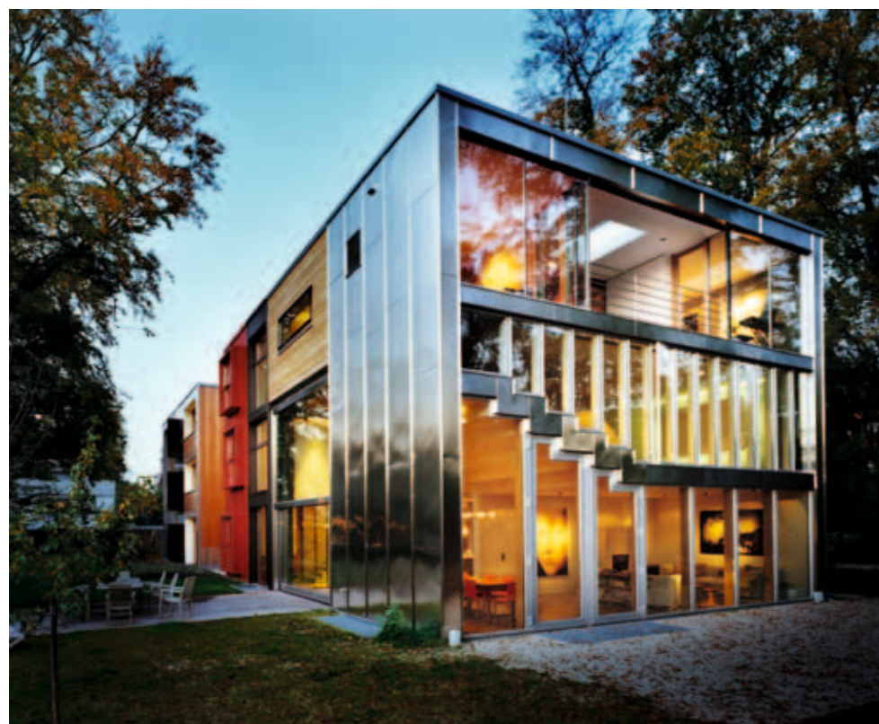
MVRDV | BARCODE HOUSE – MUNICH
